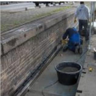
The expansion joints on the crosscut edges must be at least 1 cm wide to allow for the expansion of KLP®. This joint can be sealed.
