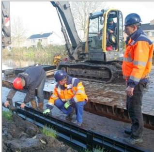
**KLP<sup>®</sup> RapidRetain System** presents a sustainable and cost efficient solution for your retaining wall! KLP<sup>®</sup> plastic is an excellent choice, especially at the water and air interface, where wood is most sensitive to rot. KLP<sup>®</sup> RapidRetain system consists of KLP<sup>®</sup> RapidRetain panels and KLP<sup>®</sup> RapidRetain combi-poles.
