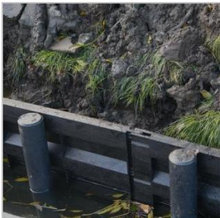
The panels are tough enough and stiff enough to be pushed into soil by crane. The KLP<sup>®</sup> RapidRetain panel coupling is made strong, so that no pole is needed directly in front of each connection. The result is that all poles can be placed in one go and subsequently the panels can be placed in one go, which translates to faster turnaround times and therefore savings.
