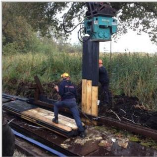
The advantages of KLP<sup>®</sup> Combi Pile Planking are that where water and air meet rotting will no longer take place and that it does not require maintenance. The result of combining plastics and wood is an extraordinarily stiff sheet piling plank. A really durable cost effective and sustainable solution. KLP<sup>®</sup> Combi Pile Planking is subject to sustainability class 1 and has a minimum technical lifetime of 50 years.
