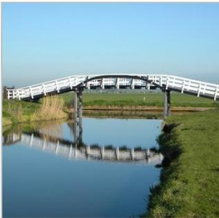
The construction consists entirely of plastics supported by the unique properties of our KLP®-S Steel Reinforced Plastic Beams. With these steel-reinforced plastic beams, it is possible to construct bridges with much larger spans. This means that, compared to traditional construction, fewer poles or beams are needed. This can lead to considerable savings on the overall material and construction costs.
