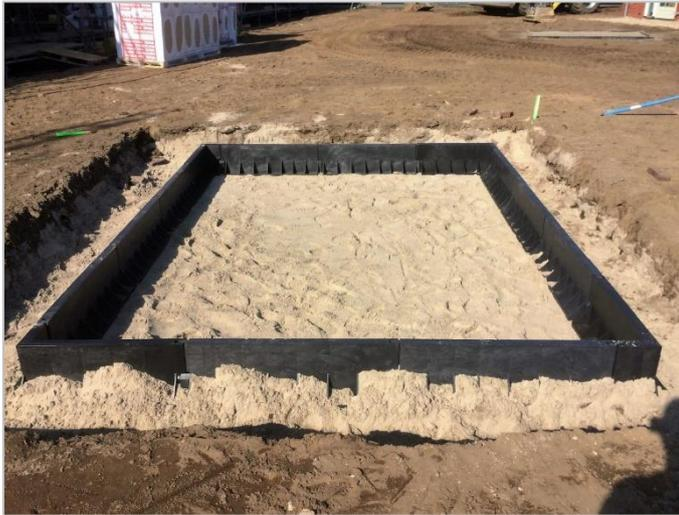
Three types of foundation block are available. All three can be connected to each other to customize your foundation.
