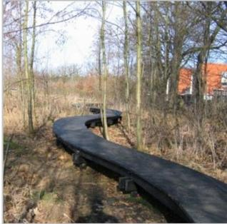
**KLP® Deck** has the charm and usability of wood plus the lifespan of plastics. This durable material will last for decades and does not require maintenance. KLP® Deck is used in platforms, walkways, balconies, bridges and jetties.
